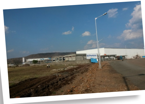
Facility view – South
