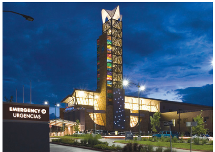
Hospital Combined Heat and Power LEED Platinum Award
