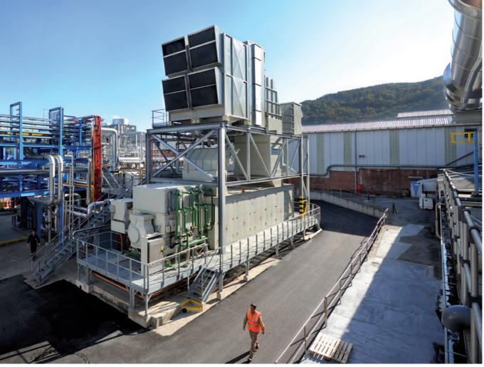
A paper company in Spain is increasing the sustainability of its production process using a 22 MWe gas turbine generator set.
