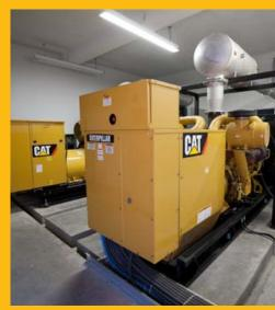
Cat<sup>®</sup> diesel generator sets supply standby power for Conduspar's factory operations and also allow the company to engage in peak shaving activities during evening hours when power is most expensive.
