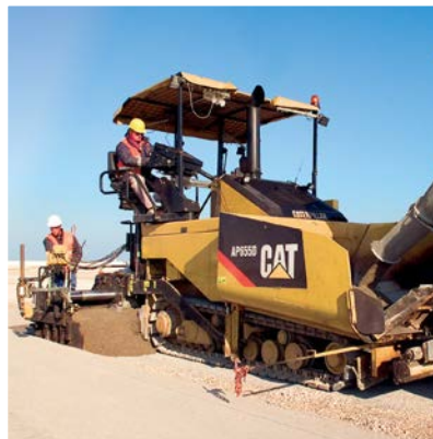
^ AP655D/AS4251C RCC Mix
