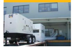
A Cat<sup>®</sup> 30-ton, 10,000 cfm chiller from NC Power was connected to a 100 kW XQ100 sound-attenuated generator on the loading dock of the Fred Hutchinson Cancer Research Center. It took NC Power just four hours to gather the equipment, transport it, set it up and get the system running when the Center's cooling system failed.
