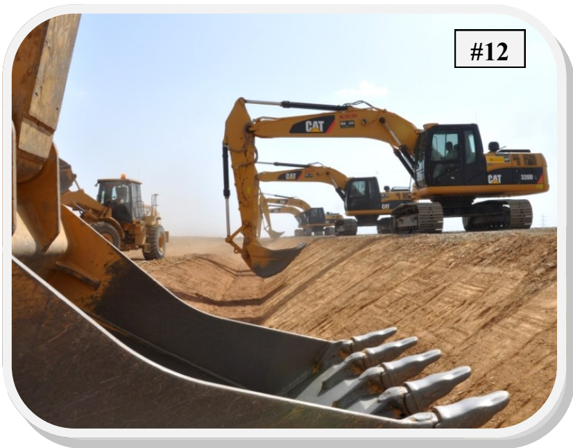
12. The 3200L Excavators are using their buckets to tamp down the dirt along this trench.
