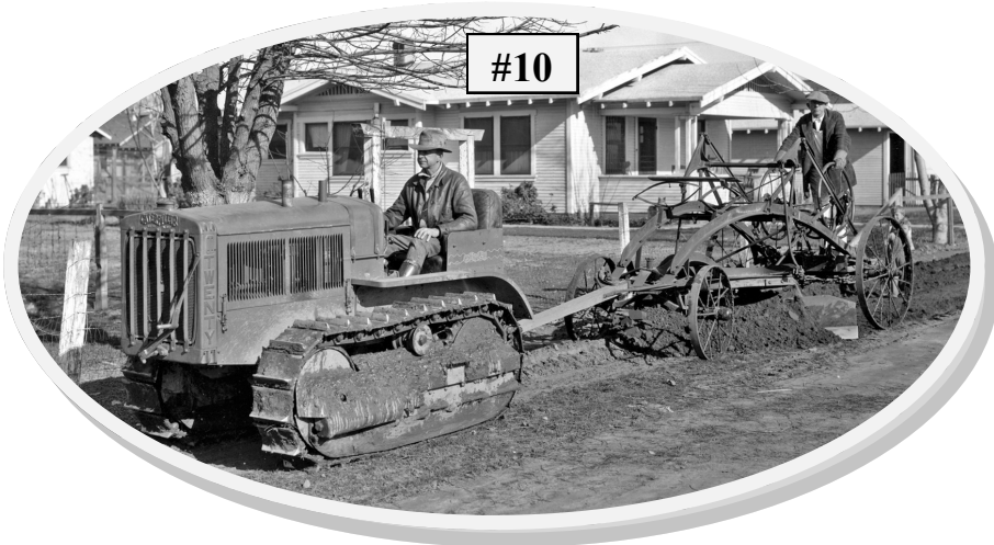
10. The scraper is attached to the back of the Caterpillar Twenty Tractor.
