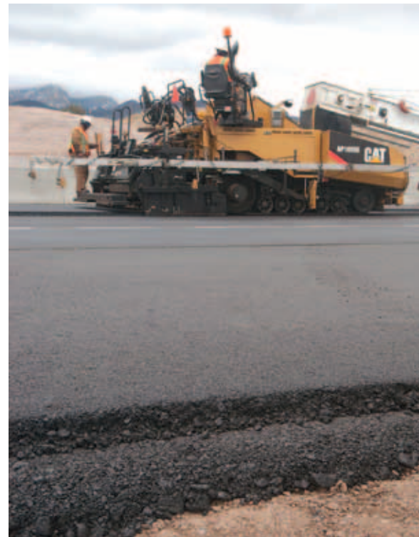
^ The crew worked from the inside to the outside to help with jobsite traffic flow.
