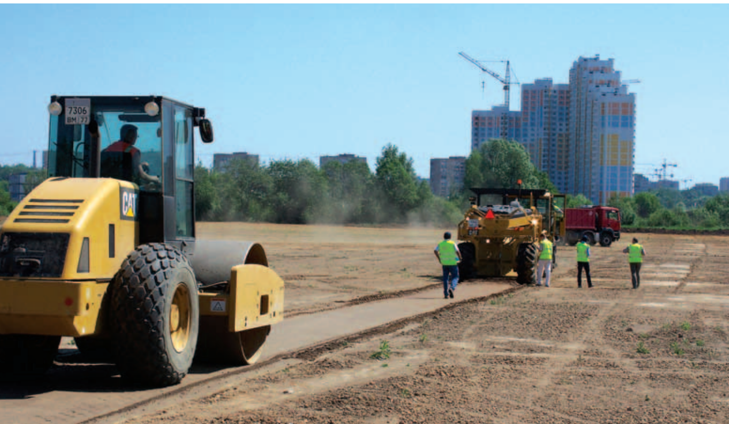
▲ The Cat RM500 Rotary Mixer on the 30 hectare site near Moscow is followed by the Cat CS533E Vibratory Soil Compactor.
