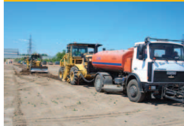
▲ A Cat Motor Grader profiles the site behind the RM500 Rotary Mixer before compaction.
