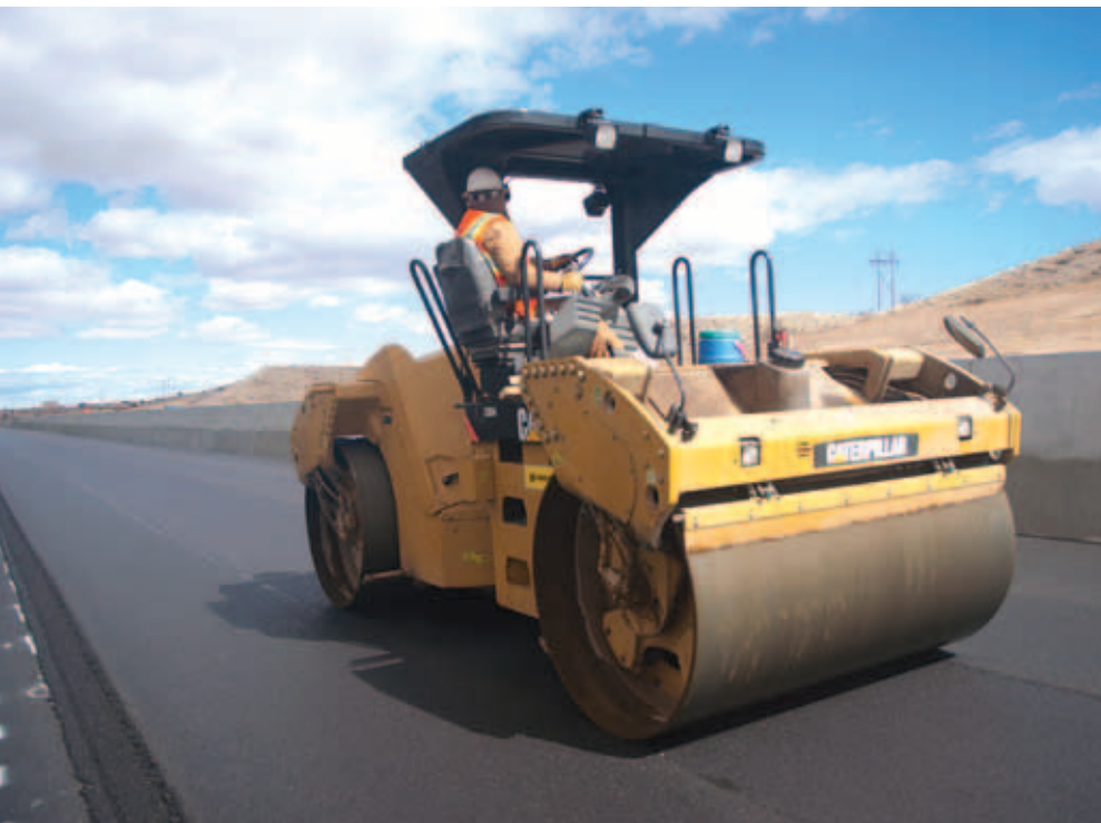
▲ The CB64 completes intermediate compaction.
