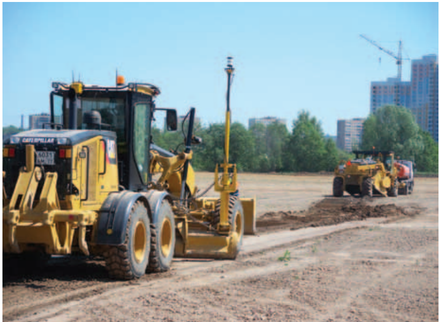
▲ The RM500 rotary mixer and its feed truck are followed by the Cat Motor Grader.
