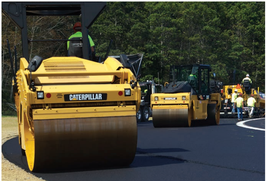
▲ The Cat® CD54 and CB54 worked next to, but never crossed over, the crown.
