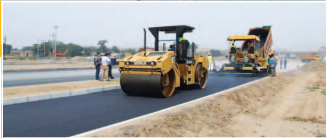
^ 2 m (79") Cat compactor working in the hottest temperature zone staying ahead of the tender zone.
