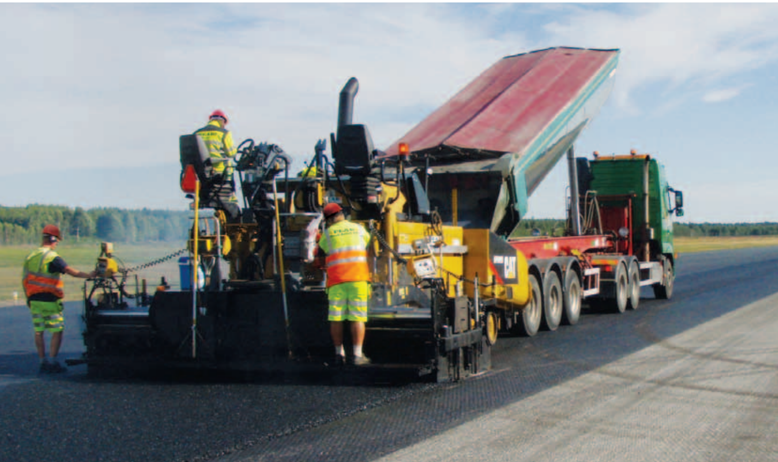
^ The paver moved at a consistent pace.
