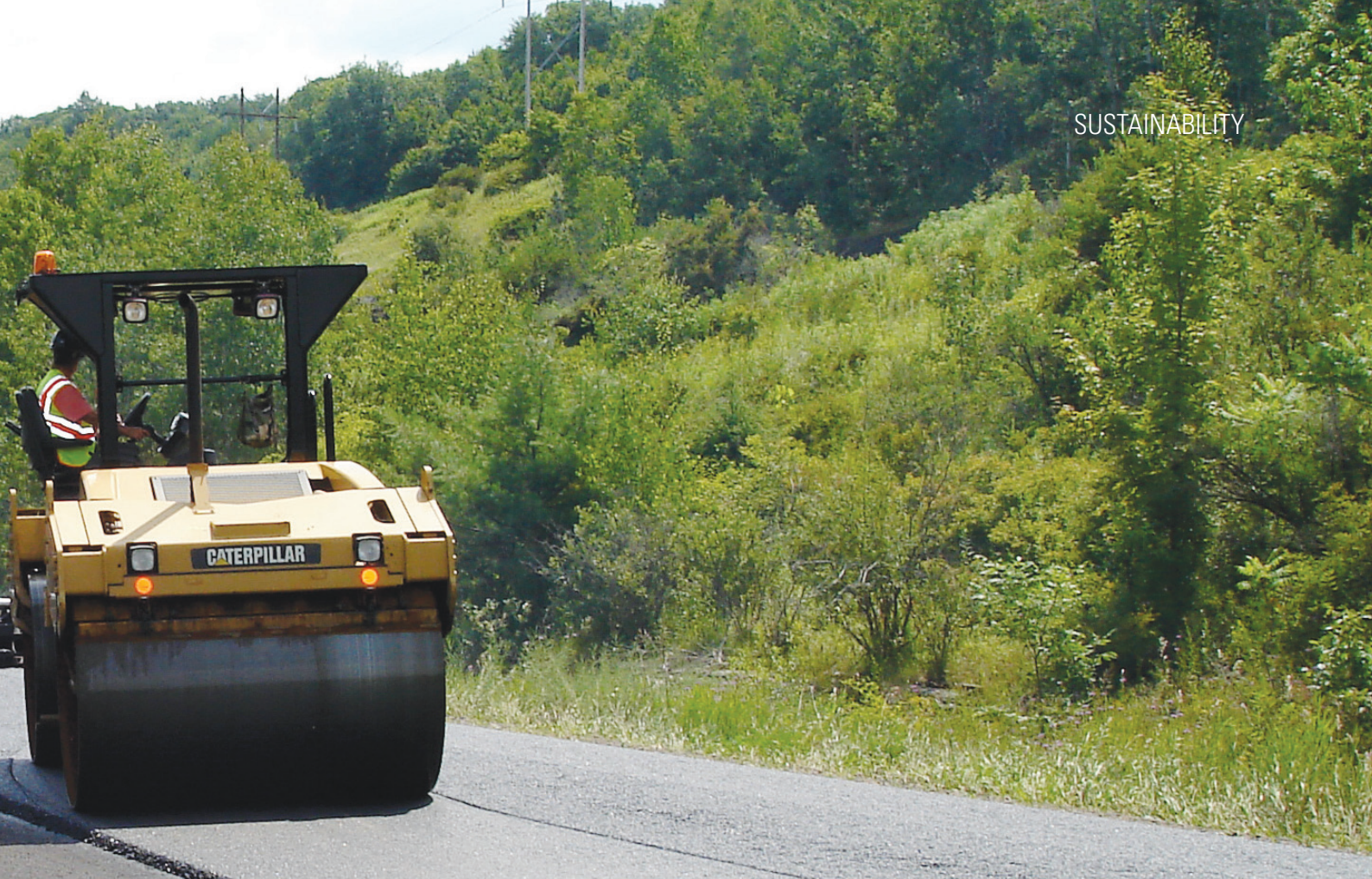
2m (79") Cat® compactor working in the hottest temperature zone staying ahead of the tender zone.
