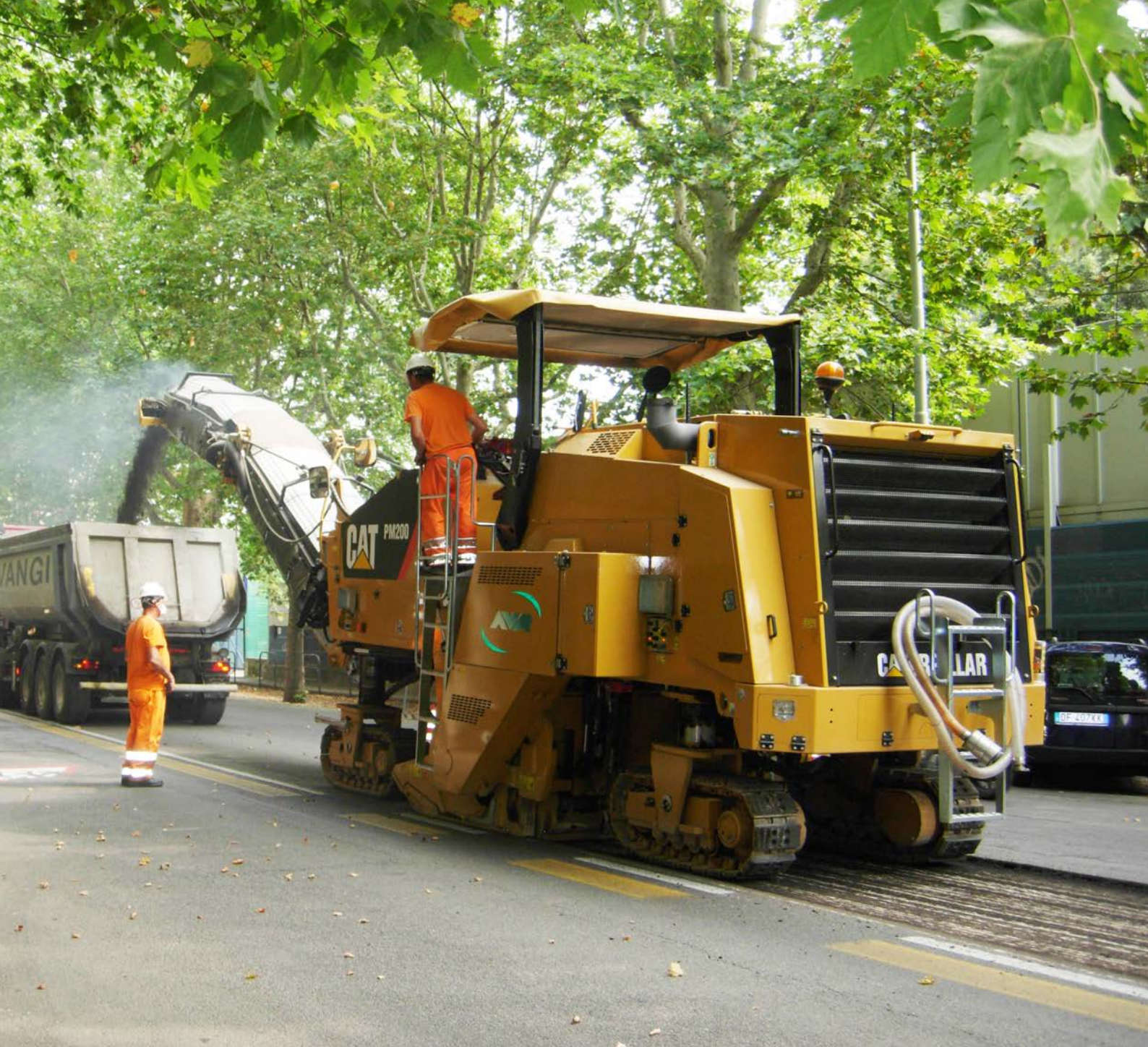
Removing the existing, damaged surface was the first step in the project. ^
